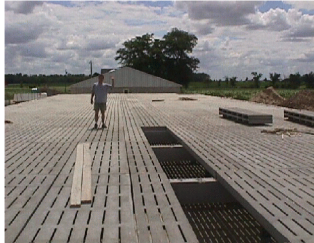
Figure 2 Slatted floor (concrete), nearly complete
